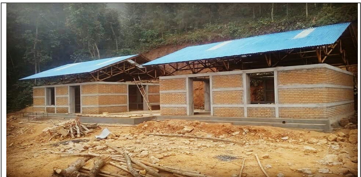
Construction is in progress
